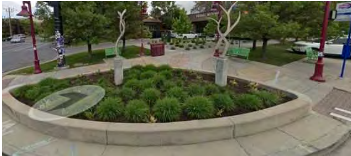
9th and 9 th Curb Extension
