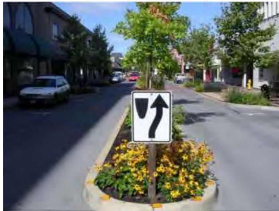
Example from Seattle of a median that functions like a choker to squeeze traffic and lower speed
