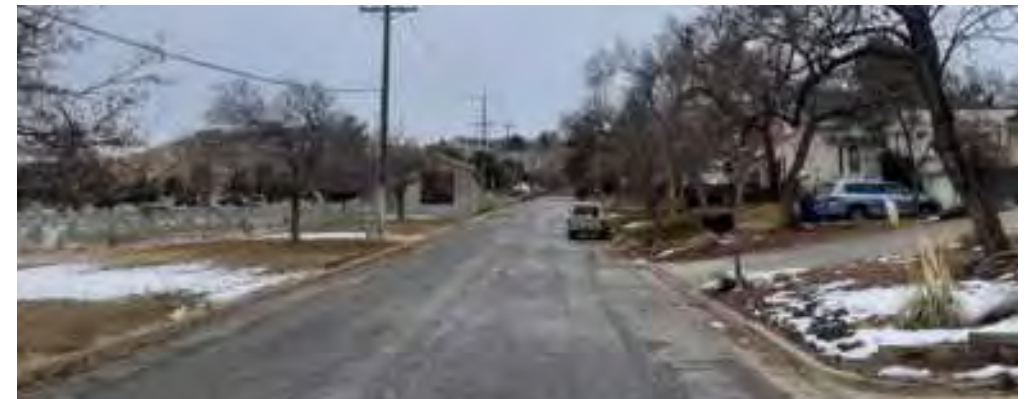
U Street with no sidewalks
